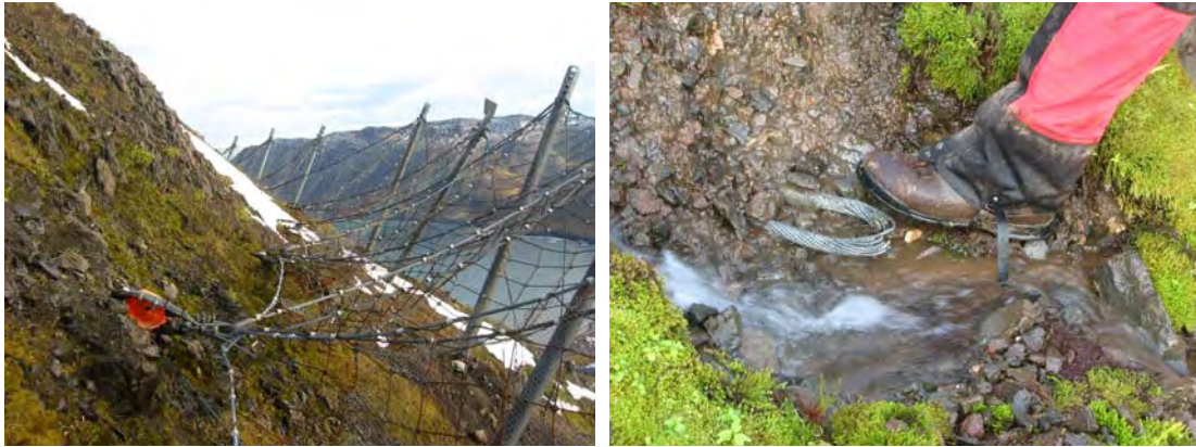
Figure 4 An instrument for measuring tension in the Geobrugg net row (left) and a broken top loop in a wire rope anchor from the same row (right).
