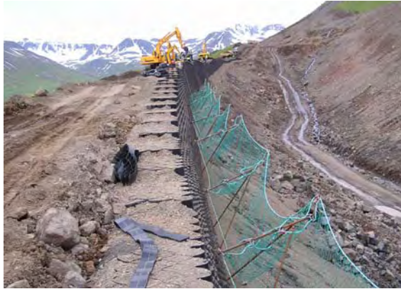
Barrier built up with geo-cells, under construction, Siglufjörður 2006.
