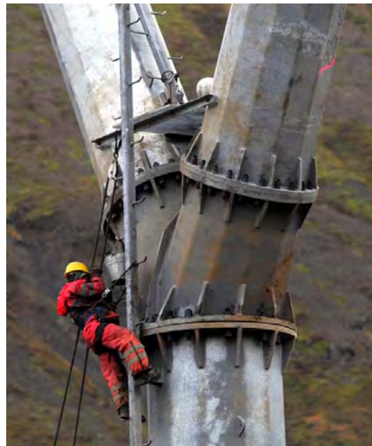
Figure 10: Main dimensions of 40m suspension tower. Figure 11: Assembly of Y connection.
