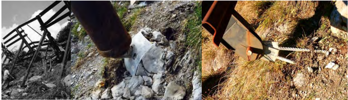
Figure 2b Damages (failure) of snow bridges (protection work in the starting zone) due to rock fall (left), slip of foundation (middle) or destruction of anchorage (right).
