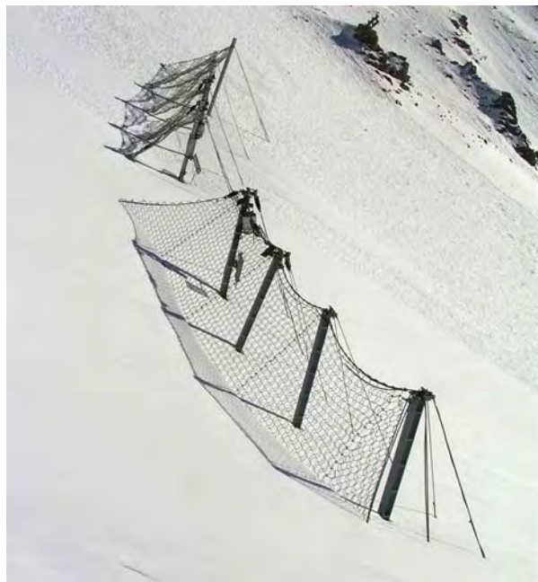
Figure 2 Rectangular snow net system in the front and triangular snow net system in the back.
