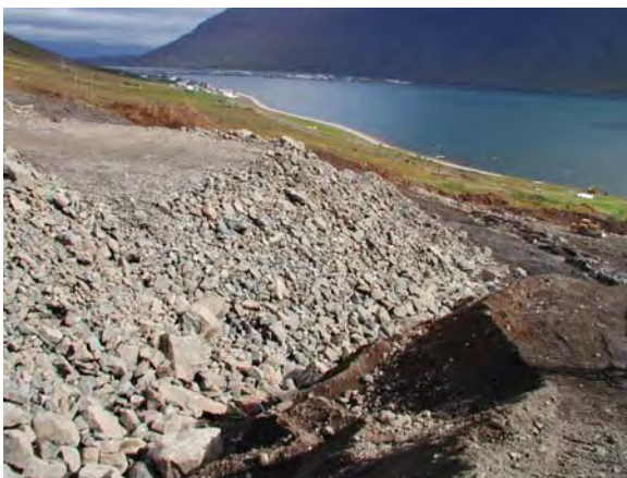
Rock fill material in deflection dam, Ísafjörður 2003.
