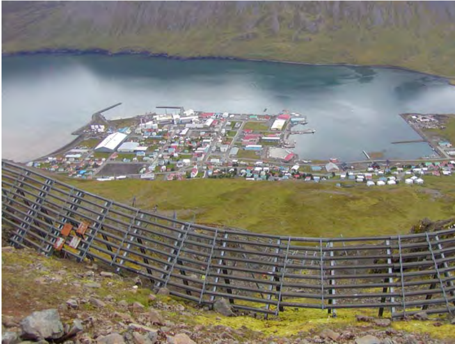
Figure 2 Uppermost row of J. Martin snow bridges. The line is adapted to the curved terrain. Plates for measuring maximum snow pressure are seen on the left side.
