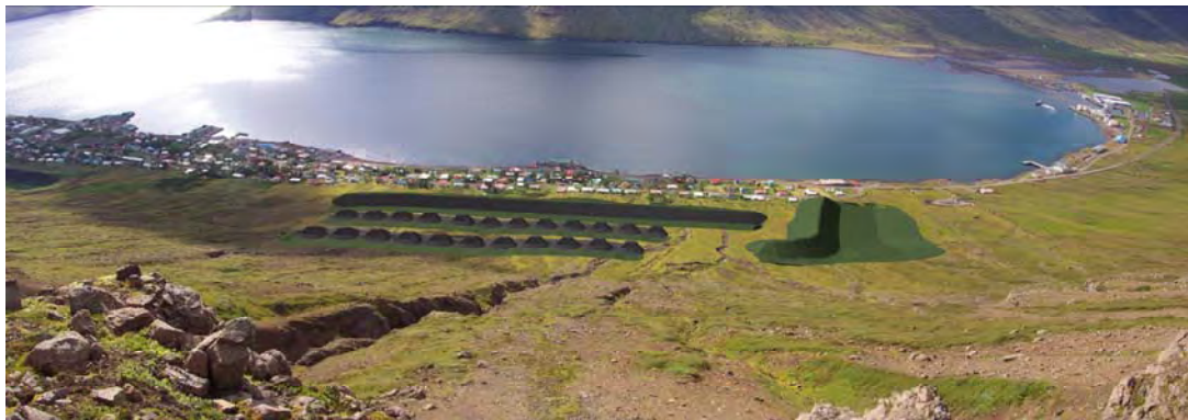
Figure 4 Proposed avalanche defences in the Tröllagil-area, Neskaupstaður. A catching dam with steep front, braking mounds and a deflecting dam (photo: Hallgrímur D. Indriðason, computer illustrated).
