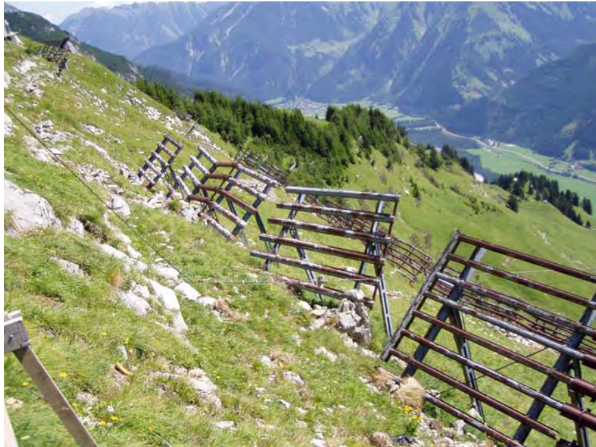
Figure 3 Steel snow bridges in an unsatisfactory condition; implemented in 1960–1970
