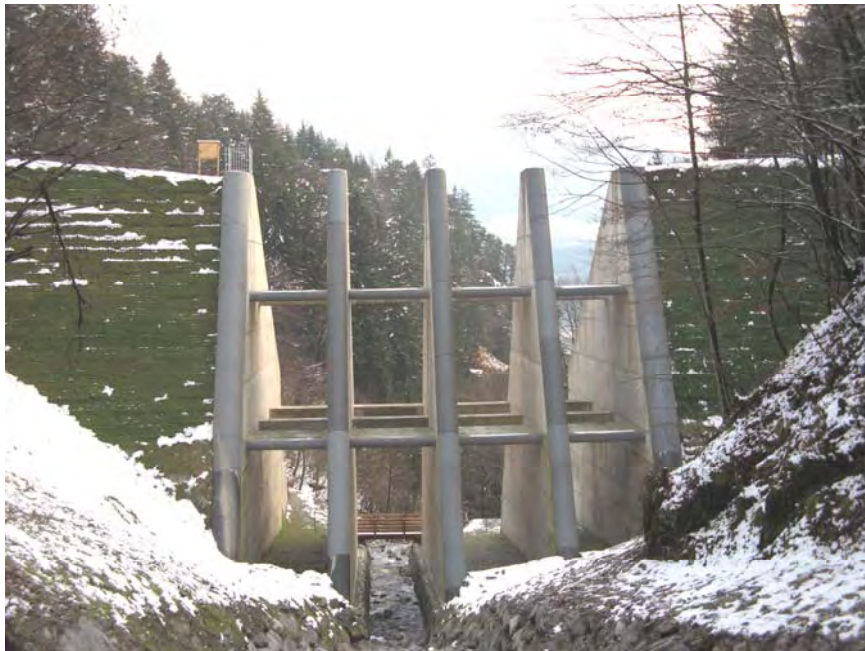
Figure 2 Braking dam at station km 1.7 (photo: Gwercher/WLV Innsbruck 2007).
