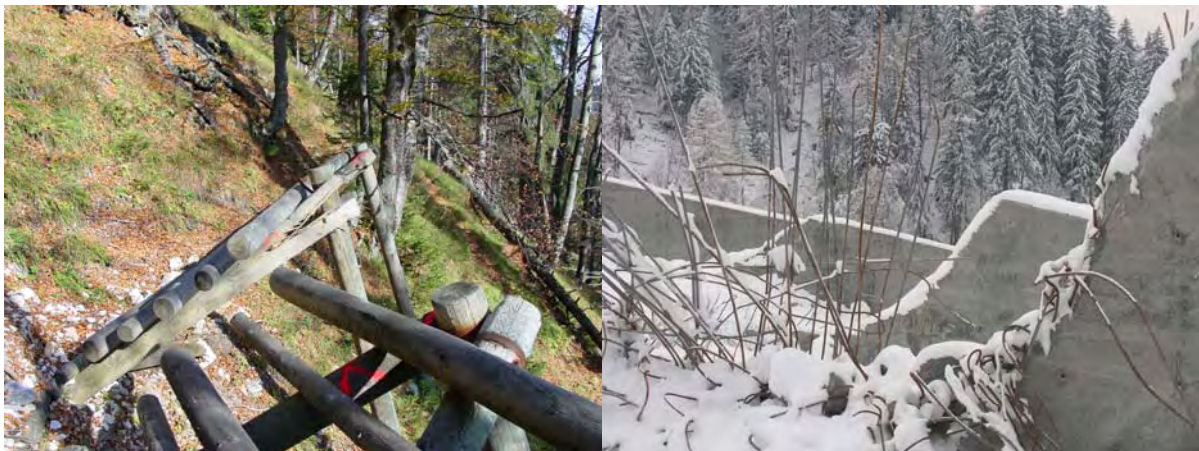
Figure 2c Damages (failure) of wooden snow bridges (protection work in the starting zone) due to collapse of the supporting construction (left); destruction of concrete retarding barriers due to extreme avalanche pressure (right).
