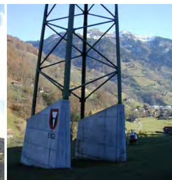
Figure 8: Avalanche tower on concrete walls
