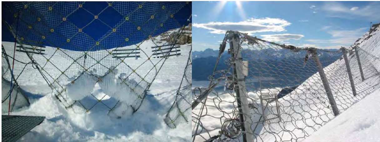
Figure 1 Detail of a Geobruigg snow net (photo on the left) and a Trumer snow net (right side), (photo: BFW).
