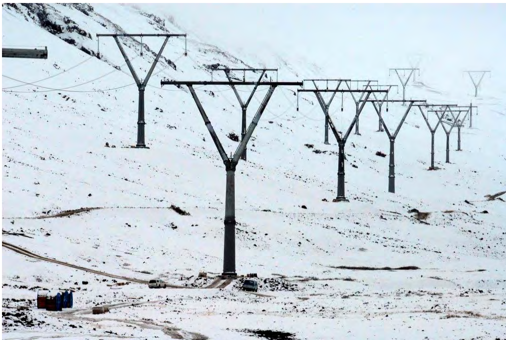
Figure 12: Avalanche towers in Áreyjardalur, spacing between lines is 60m.
