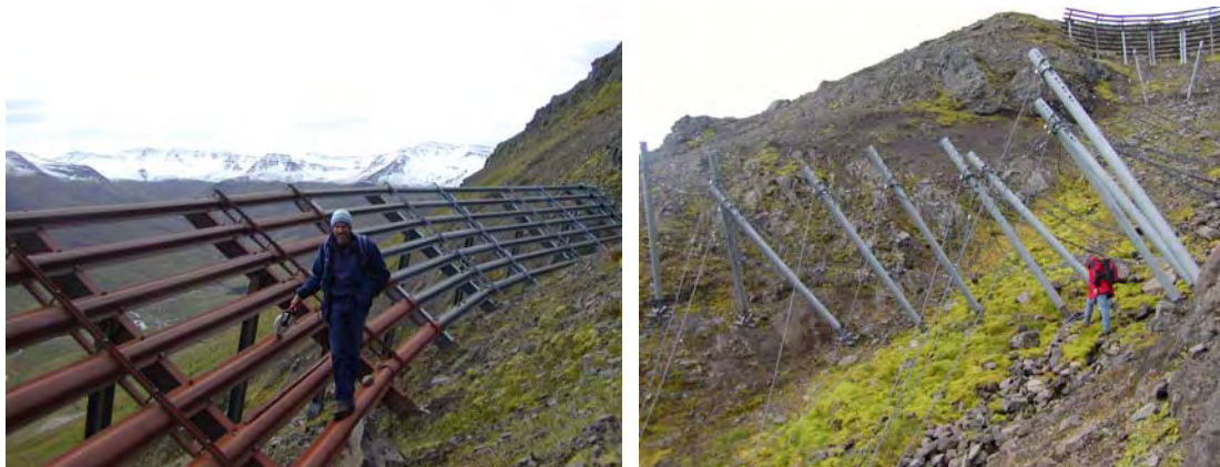
Figure 7 Comparison of galvanized and black type of snow bridges in the lowest row of the J. Martin snow bridges (left). The row with EI snow nets was deformed by the heavy snow loads, partly due to lack of lateral stability.
