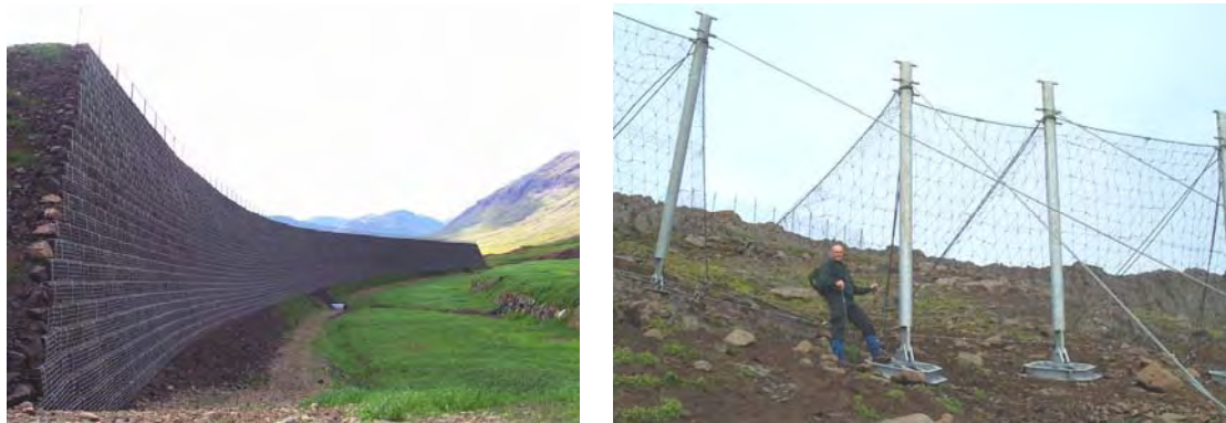
Figure 3 Avalanche defences in Drangagil, Neskaupstaður. Catching dam with steep front and supporting structures (photos: Hallgrímur D. Indriðason).
