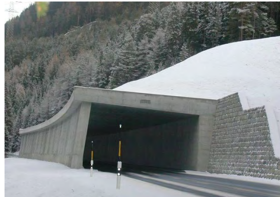
Figure 2 130 m long snow shed built at Val Raschtsch in 2002 as a monolithic jointless concrete structure.
