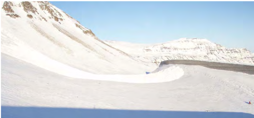
Figure 1 A catching dam at Brún in Bjólfur in Seyðisfjörður, eastern Iceland. An avalanche that fell on the 9 th of February 2008 and stopped on the dam face can be seen. The dam is 20 m high with a 10 m high very steep upper part. (Photo: Emil Tómasson.)
