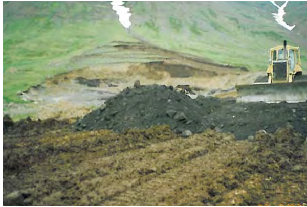
Sand being laid out on top of scree material, Flateyri deflection dam, 1997.
