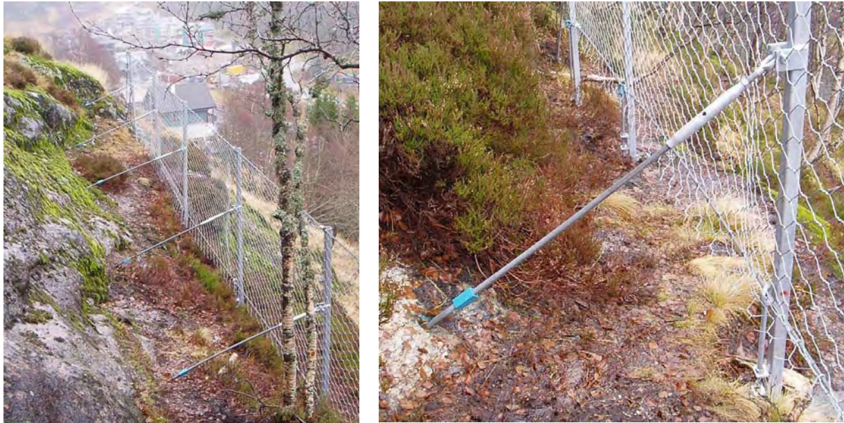
Figure 2 a) Light retention mesh. b) Strut (tread bar) coupled to rock anchor and post. Mesh with ground clearance clipped to wire going through the adjusting eye bolts.
