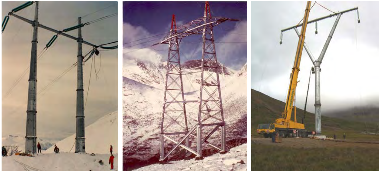
Figure 4. Different types of “avalanche” masts, to the left the French type used in Western Norway, in the middle a local type used in Western Norway and to the right the erection of one of the avalanche towers in Áreyjadalur (photo: Línuhönnun 2006).
