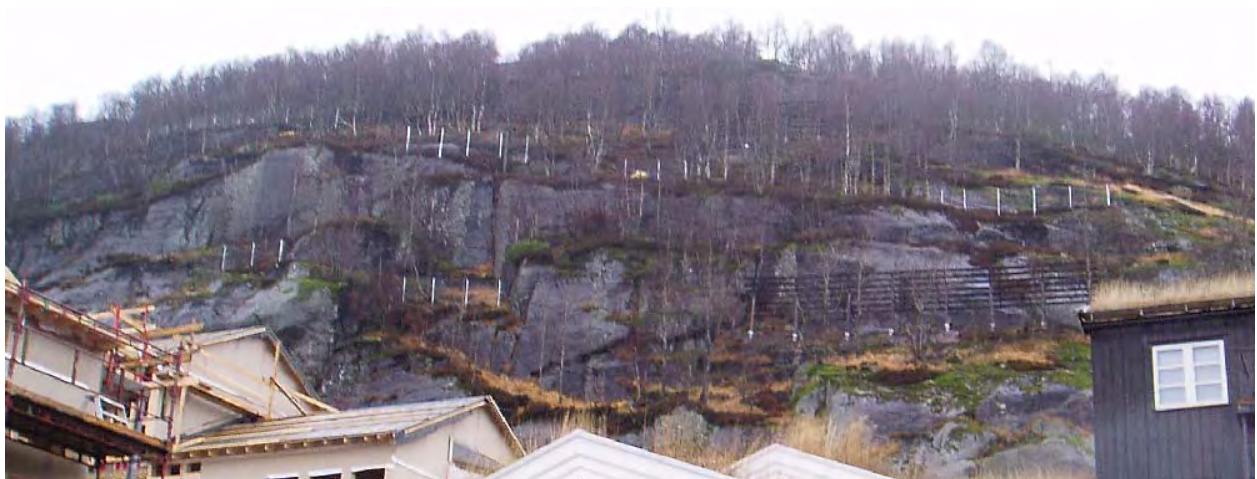
Figure 1 Tourist resort protected by light retention meshes and conventional snow bridges. Six locations of meshes can be identified by grey posts in the hillside.
