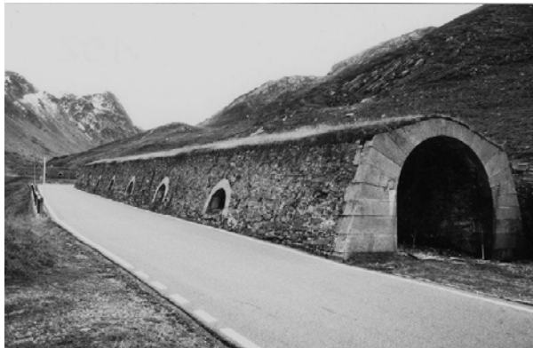
Figure 1 312m long stone-arched snow shed built at Splügenpass in 1843. The snow shed was in operation until 1950.
