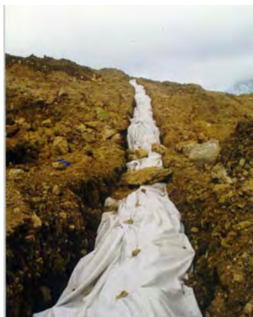
Drainage trench, Siglufjörður, 1999.
