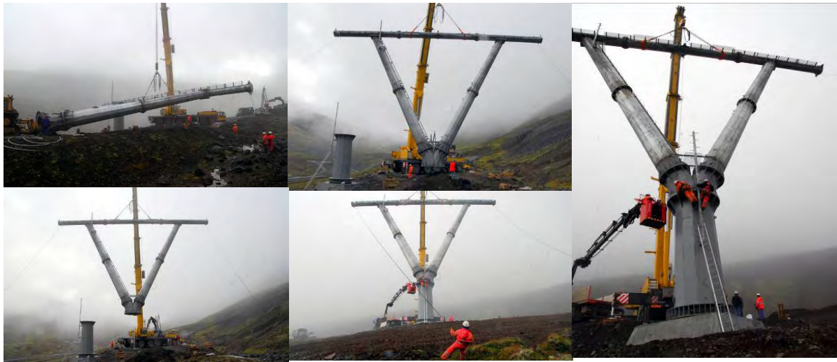
Figure 16. Assembly of upper part of tower by crane.
