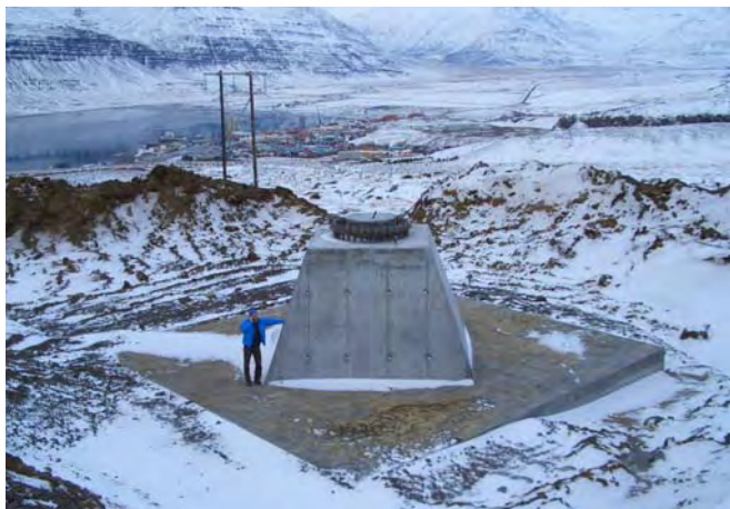
Figure 14: Foundation of Y tower.
