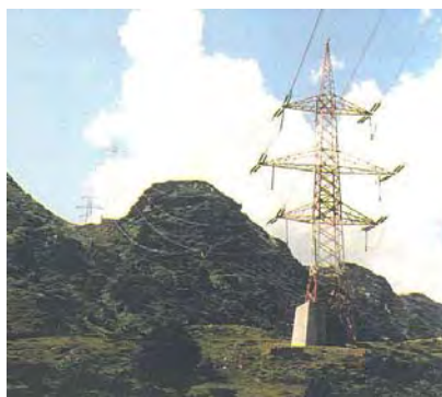
Figure 7: Tower with concrete plow
