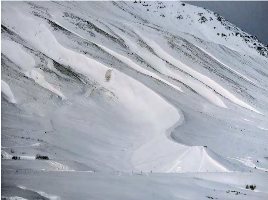
“Stóri boli” deflecting dam in winter – A well designed extension of the mountain to protect the nearby village of Siglufjörður. This dam has already deflected several avalanches away from the settlement.
