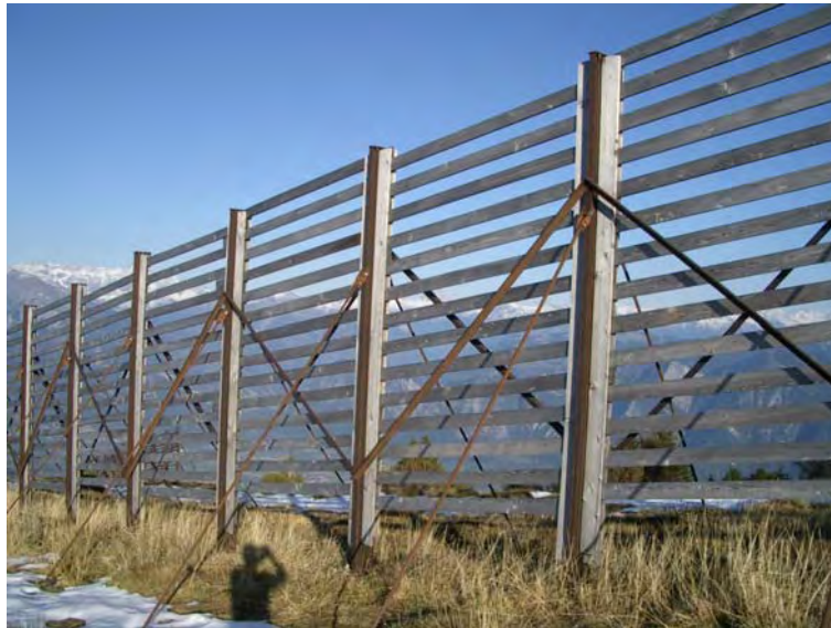
Figure 1 A 4 m high snow drift fence in Switzerland with a porosity of 50 %. The structure consists of steel posts and wooden boards. The fence is founded using ground anchors. Note that the bottom gap helps to reduce snow deposits close to the fence.
