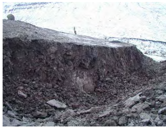
Rock cut at Ísafjörður deflection dam, Ísafjörður 2003.
