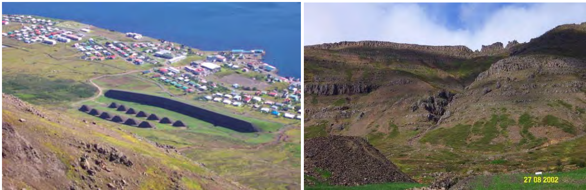
Figure 2 Braking mounds and catching dam in the Drangagil area in August 2002.
