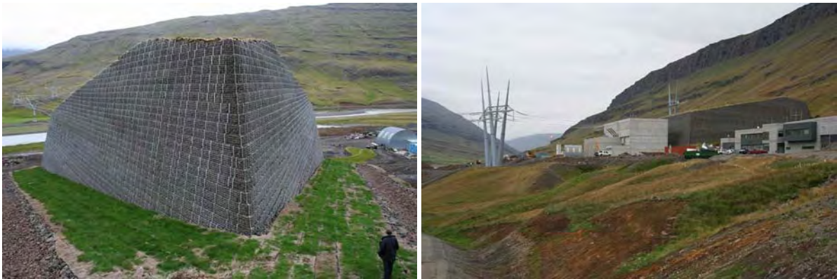
Figure 4 The splitter above the switchgear house in Fljótisdalur, during construction.
