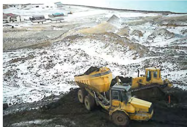
Scree material being laid out, Flateyri deflection dam, 1996.
