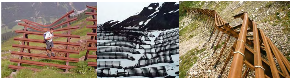
Figure 2a Damages (failure) of snow bridges (protection work in the starting zone) due to overload caused by snow pressure (left), overload due to avalanches (middle) and insufficient slope stability (right).
