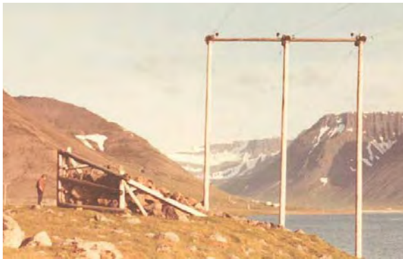
Figure 4: Plow in front of a tower in a 132 kV line. Figure 5: Avalanche tower in a 33 kV line.
