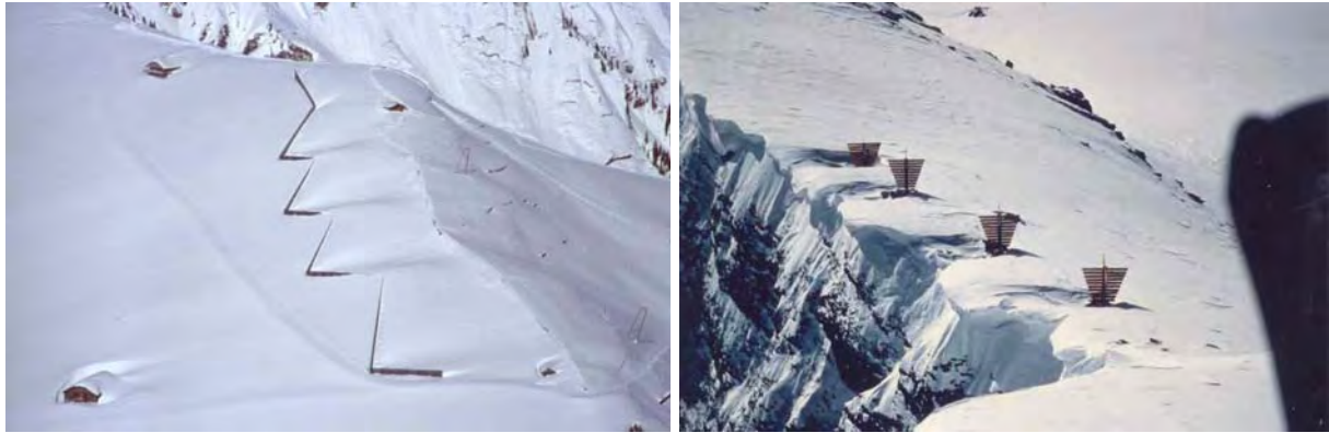
Figure 2: Snow fences to the left and wind baffles to the right in use in Switzerland (photos: Stefan Margreth).
