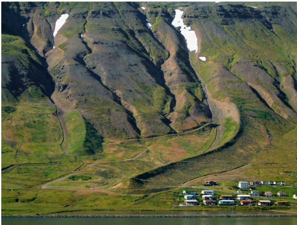
Deflecting dams, “Stóri-boli” and “Litli-boli”, near the southern end of the settlement.
