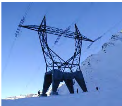
Figure 6: Avalanche tower in Switzerland
