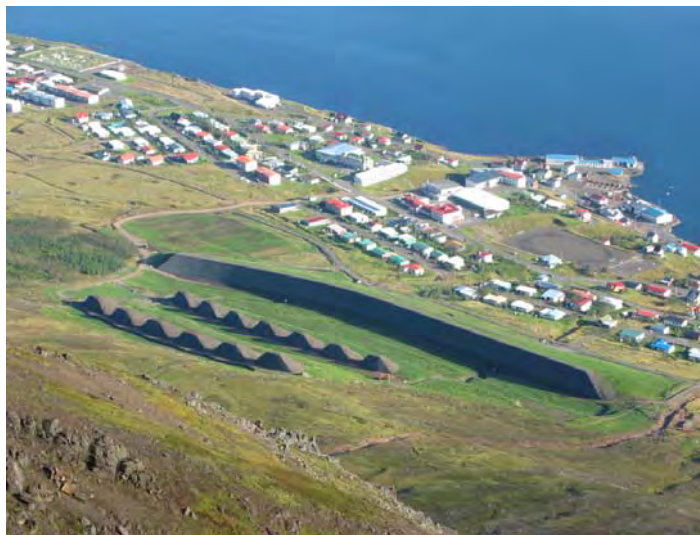
The 17 m high catching dam and two rows of 10 m high braking mounds above the settlement in Neskaupstaður.
