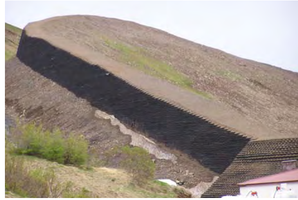
Barrier built up with geo-cells, after completion, Siglufjörður 2006
