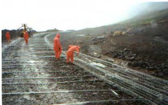
Barrier built with steel mesh systems under construction, Neskaupstaður 2000..
