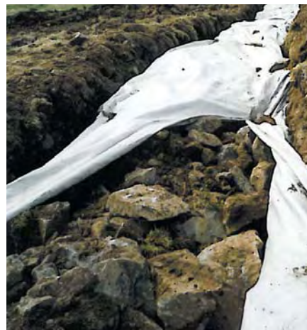
Drainage trench, Flateyri, 1997.
