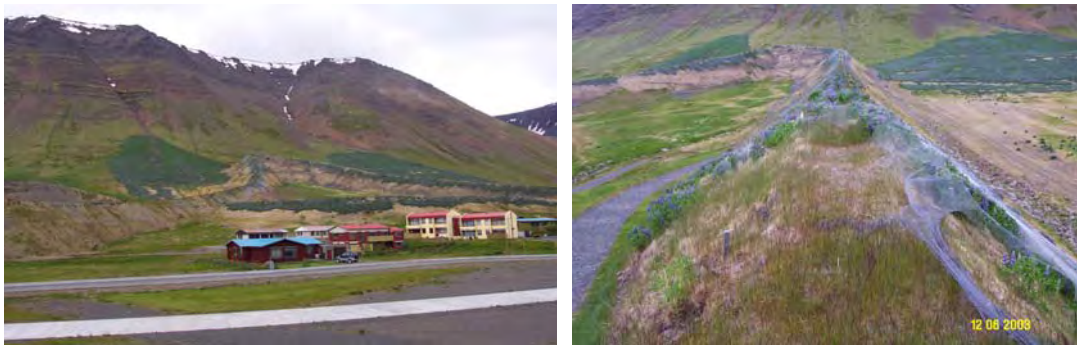
Figure 1 Avalanche defences in Flateyri. The dams are completely covered with vegetation (photos: Hallgrímur D. Indriðason).
