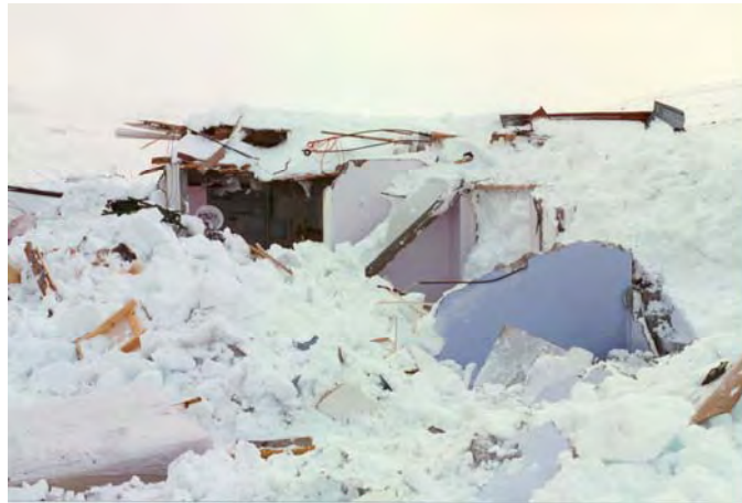
Figure 1 A house damaged by the avalanche at Súðavík on 16 January 1995.
