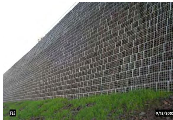
Barrier built with steel mesh systems, after completion, Neskaupsstaður 2002
