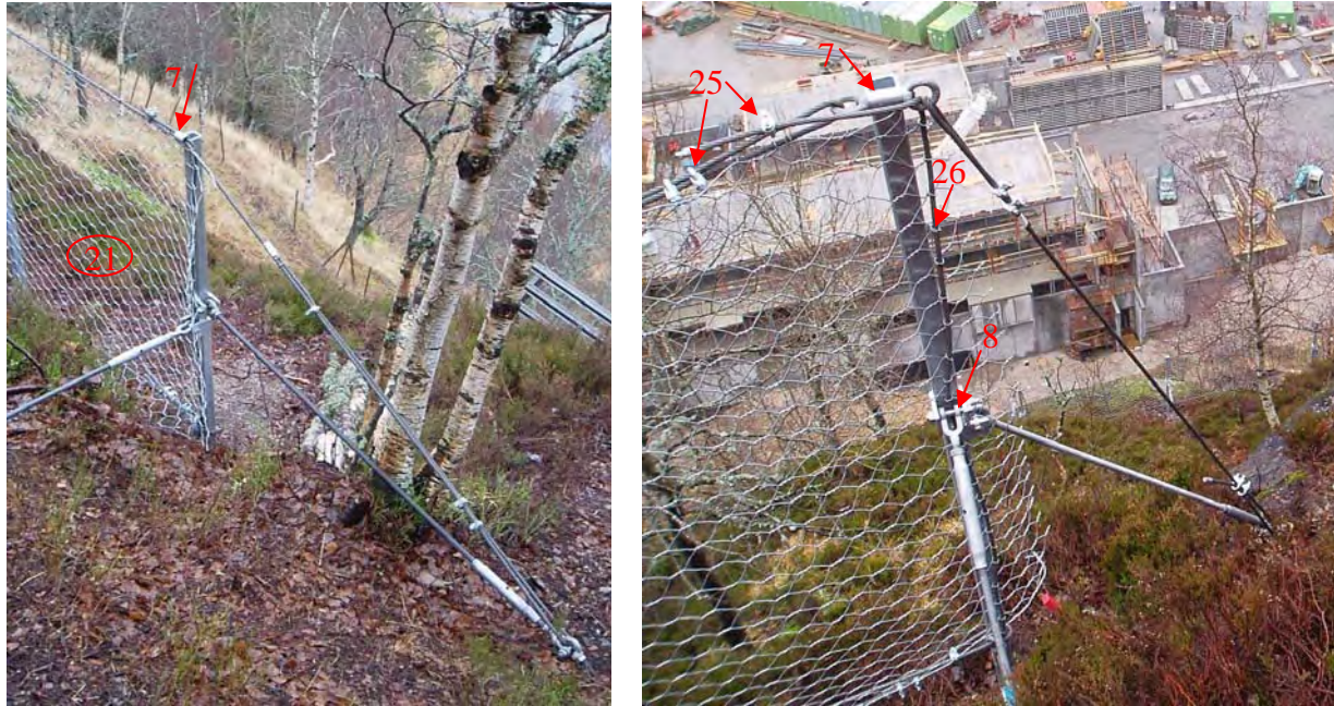
Figure 5 The bearing top wire of the mesh goes through a cable eye to the rock anchor.
