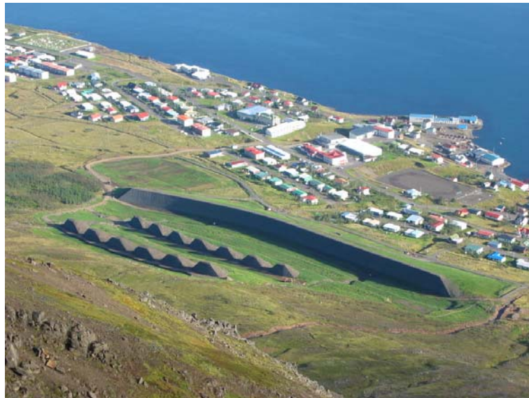
Figure 8. The braking mounds and the catching dam in Neskaupstaður. Each mound is 10 m high and the catching dam has a height of 17 m. Photo: Tómas Jóhannesson.
