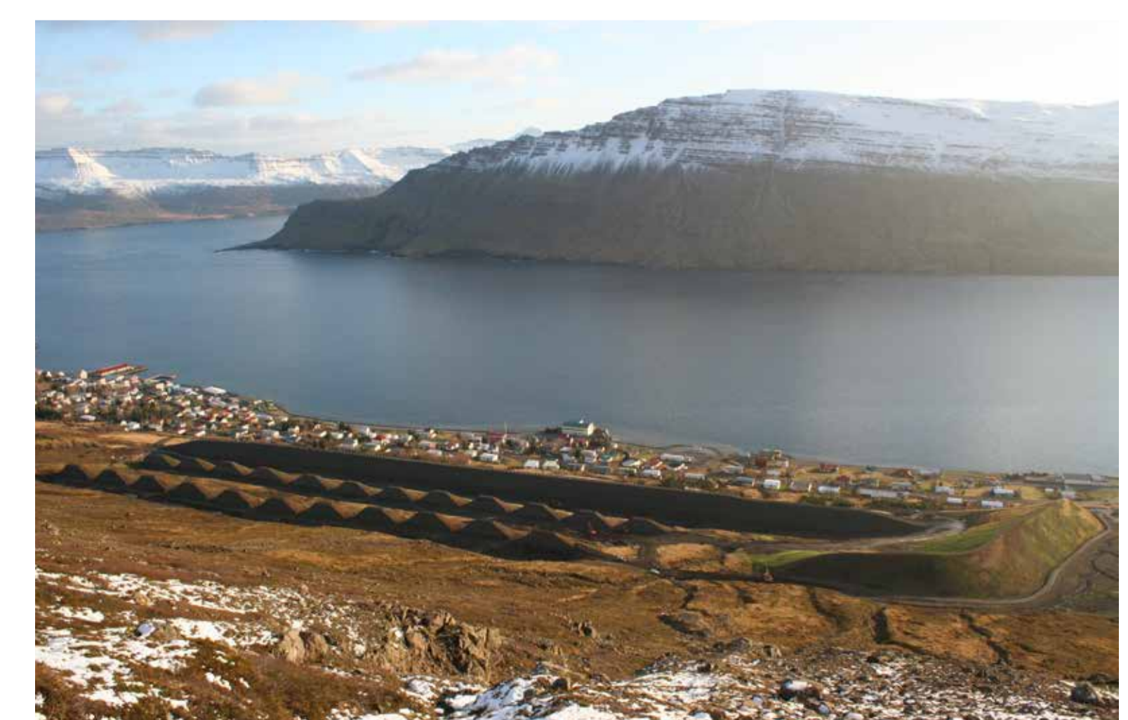
Figure 5. Catching dam, deflecting dam and braking mounds in Neskaupstaður, E-Iceland.
