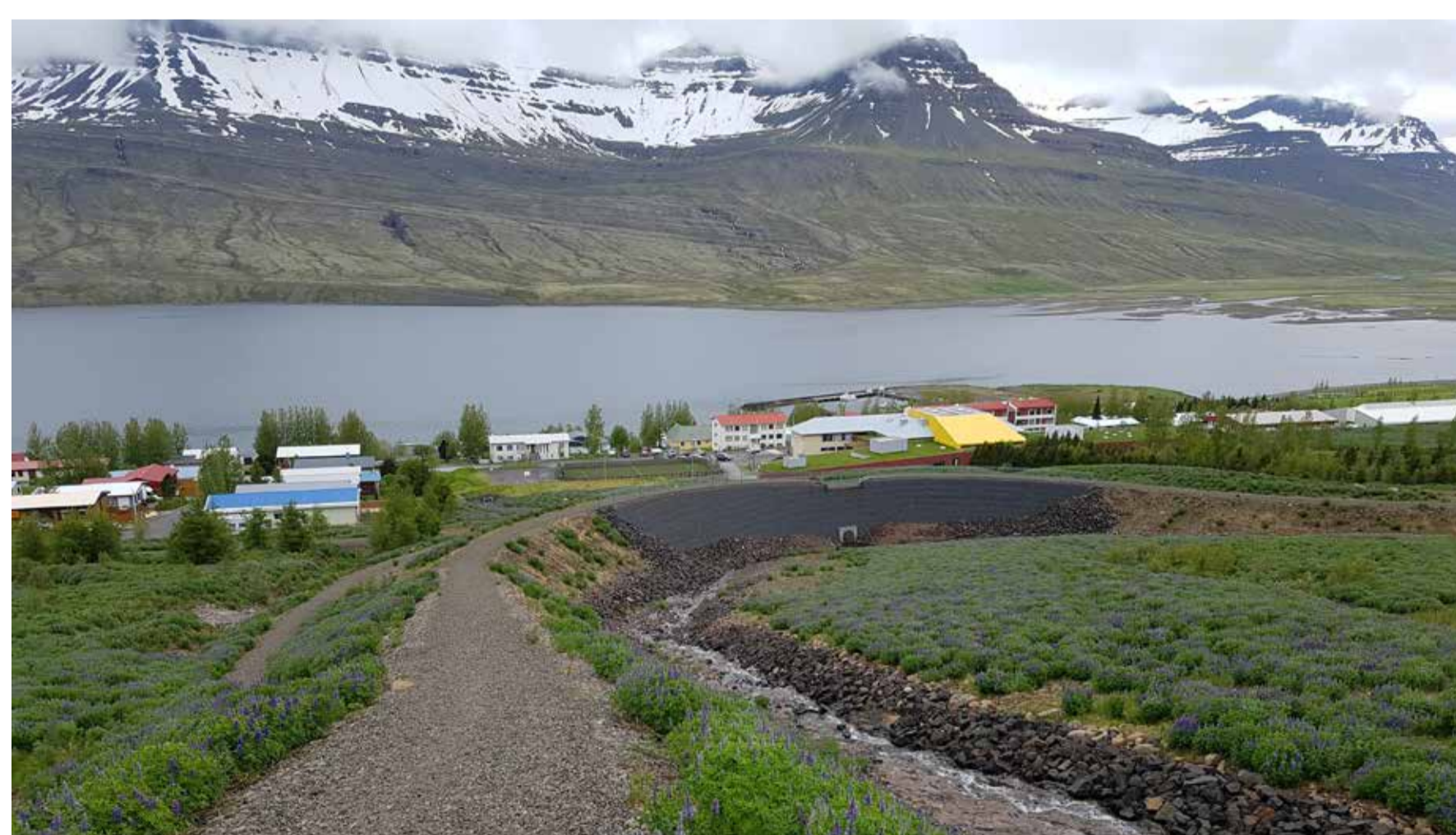
Figure 2. Slushflow protecting measures in Fáskrúðsfjörður, E-Iceland.
