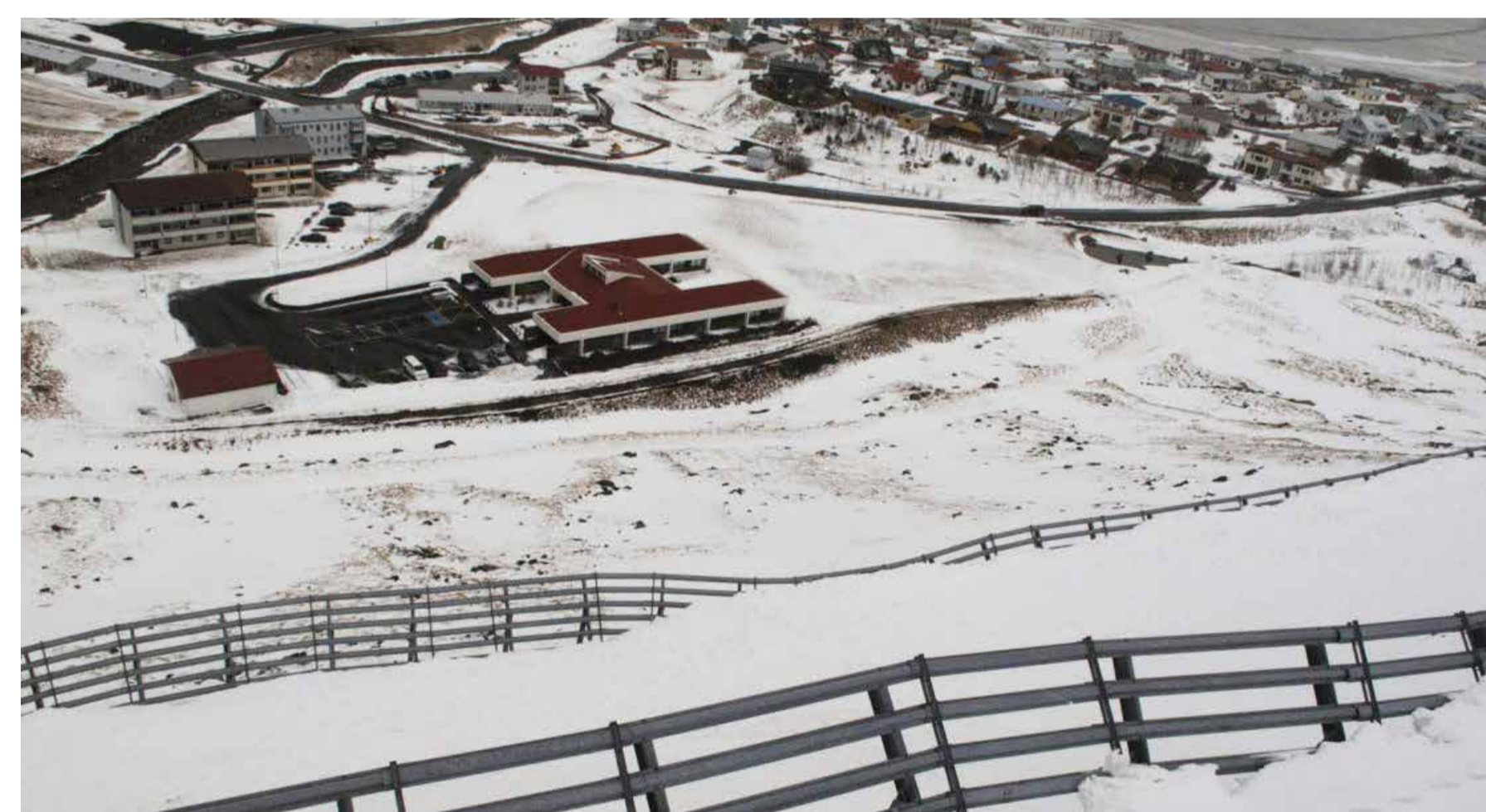
Figure 2. Supporting structures in Ólafsvík, W-Iceland.
