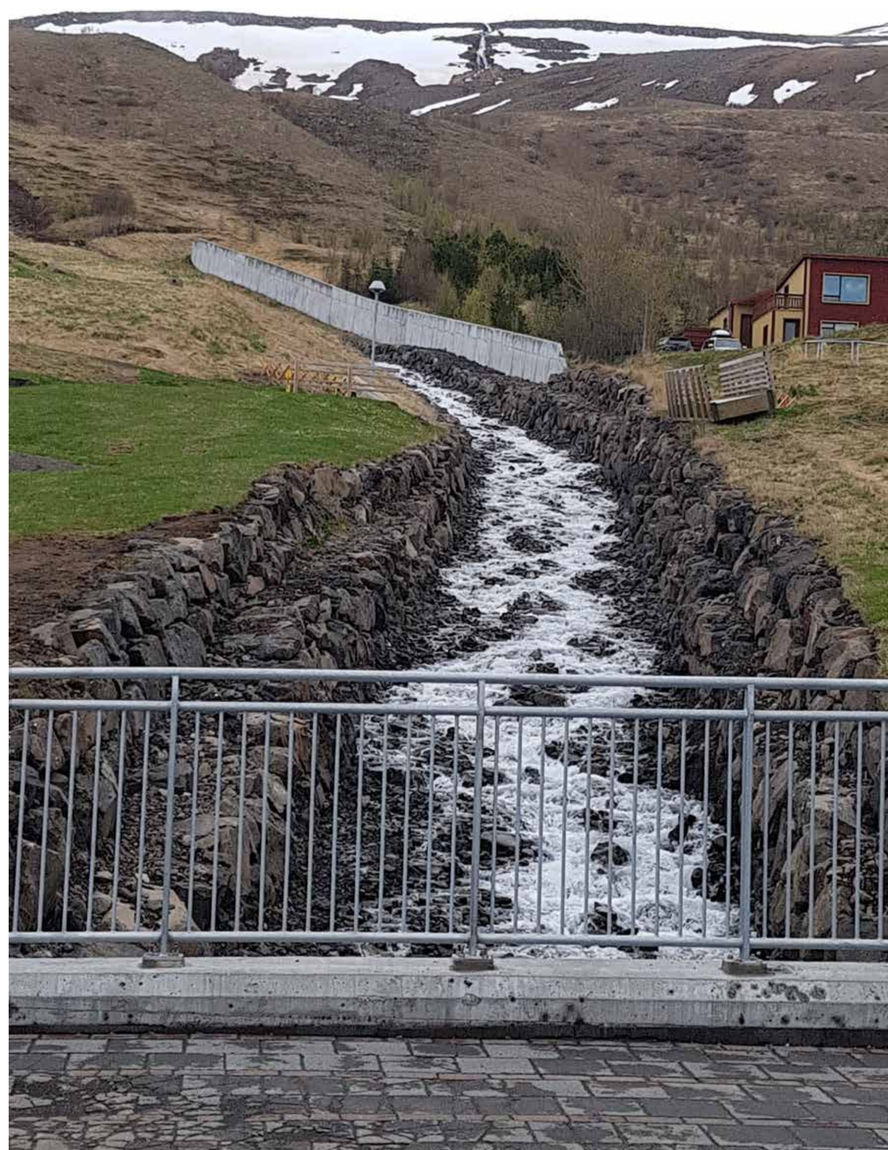
Figure 1. Slushflow protection measures in the river Hlíðarendá in Eskifjörður, E-Iceland.
