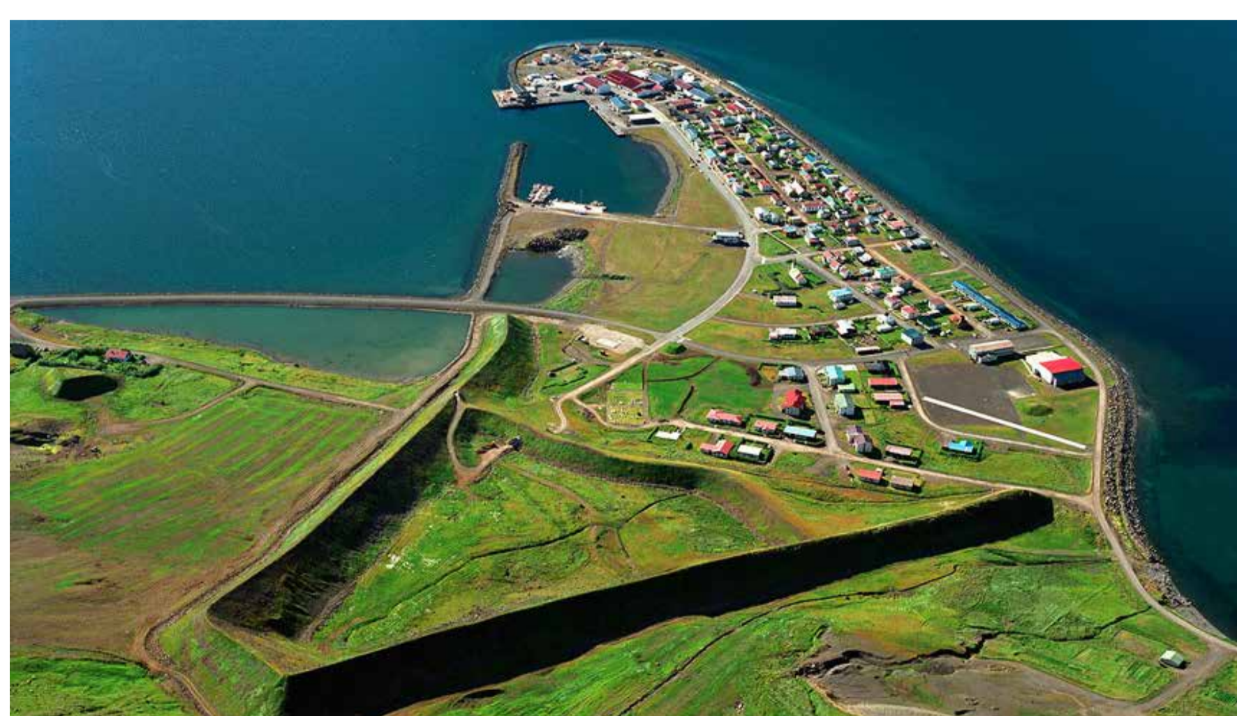
Figure 3. Deflecting dams at Flateyri, W-Iceland.
