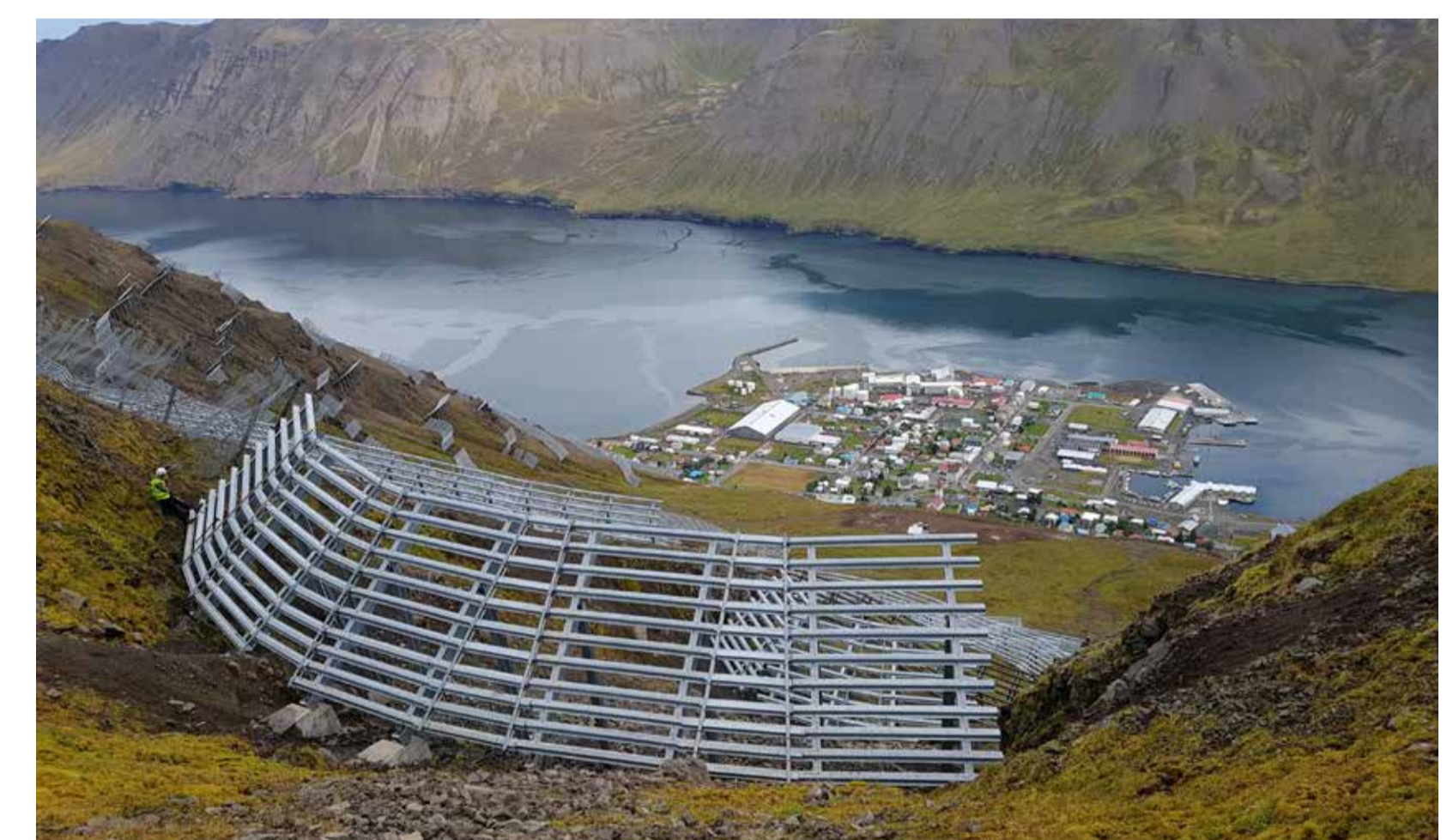
Figure 3. Supporting structures in Siglufjörður, N-Iceland.
