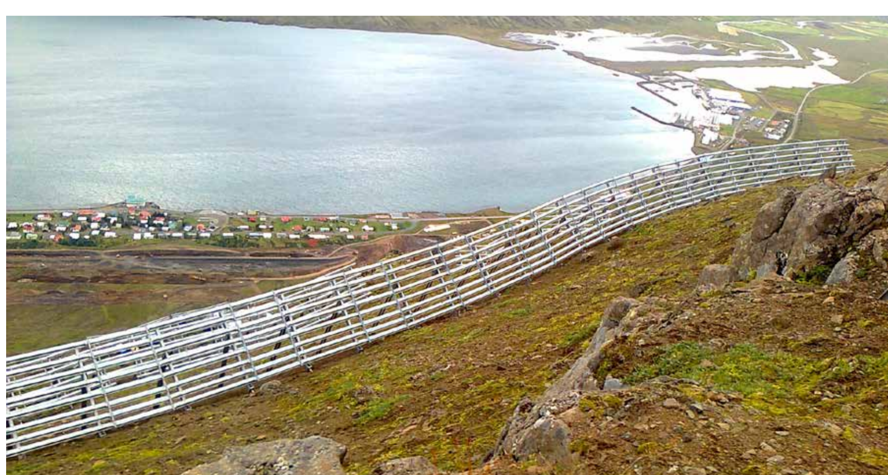
Figure 6. Supporting structures in Neskaupstaður, E-Iceland.
