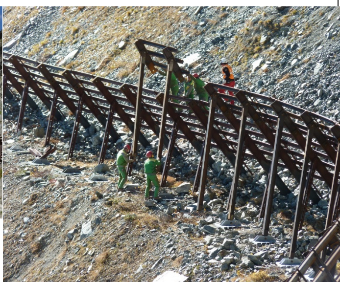
Figure 5: Construction Type flexible
