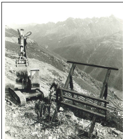
Figure 1: Installation of a supporting structure with a height of 3.5 meters, the foundation will be fixed with a concrete base and will be filled with soil material.
