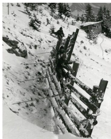
Figure 6: "Snow-hanging bridges", D_k = 3\text{m} , mounting after snowfall in the 60s of the last century in the avalanche starting zone of the Hüggen avalanche [Source: WLV Vorarlberg]
