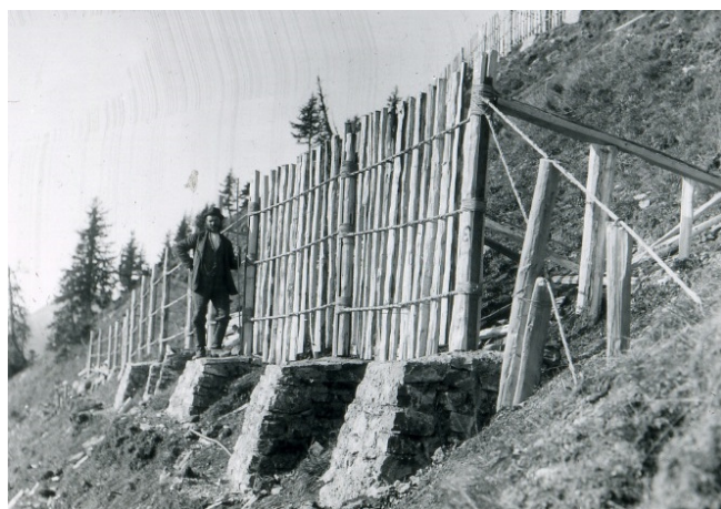
Figure 5: Arlberg Rake in the avalanche starting zone of the Hüggenlawine in the year 1906 [source: WLV Vorarlberg].
