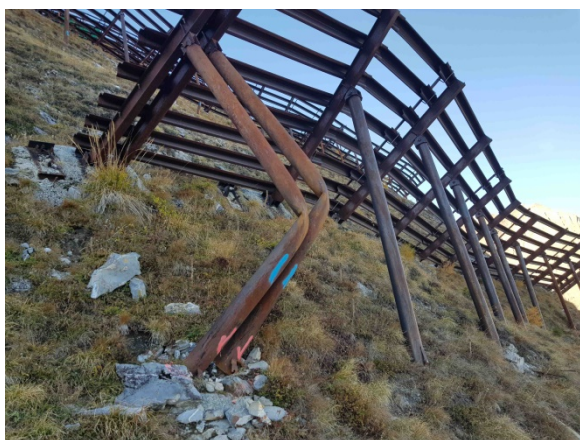
Figure 3 Buckled supports of end of line structures in the Valais. No lateral snow pressure was considered in the design (Photo Nivalp SA, 2018).
