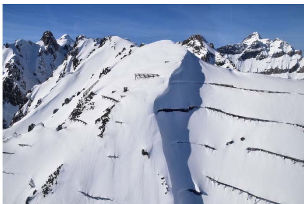
Figure 1 Supporting structures in the Valais, in the centre the structure height is 6 m. On 24 January 2018 the snow height was locally > 8 m (Photo J.J. Lugon).
