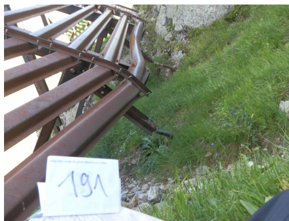
Figure 4 Deformed crossbeams and anchors because of a too large gap between lowest crossbeam and ground, canton Uri (Photo R. Planzer, 2018).
