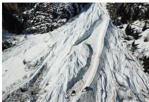
Figure 6 Deflecting dam made of snow, canton Valais (Photo W. Gitz, 2018)
