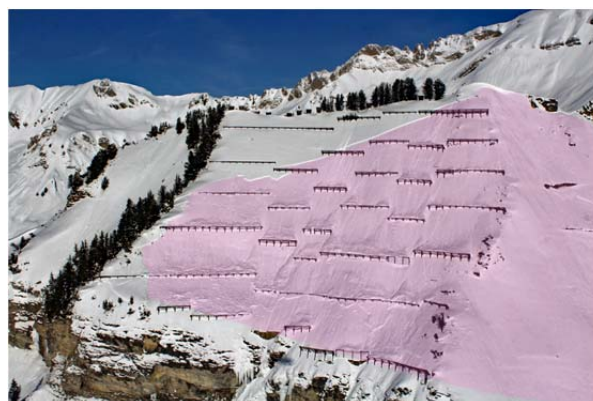
Figure 2 Supporting structures in the Bernese Oberland, on 22 January 2018 a large slab avalanche released within the controlled area (Photo U. Ryter).
