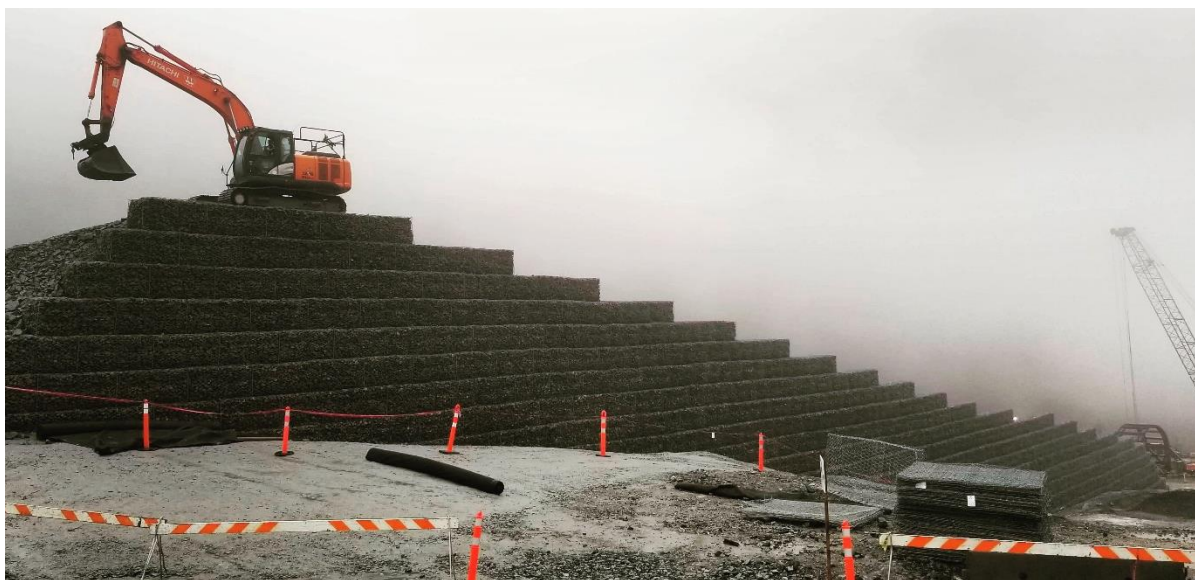
Figure 3 Final construction of the avalanche stopping wall (November, 2018).
