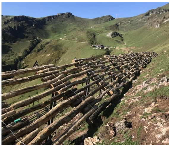
Figure 3: Support structure to protect the valley station built in the release area AG 03 (KitzSki, 2019)
