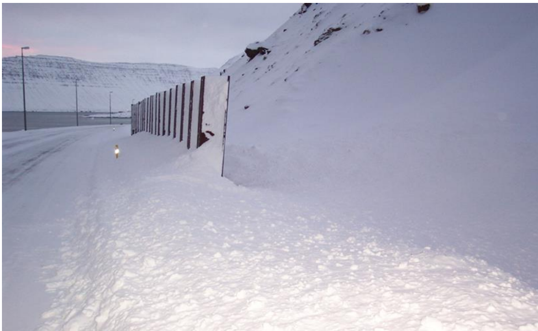
Figure 2. Steel bulkhead by the road below Óshlíð between Bolungarvík and Hnífsdalur.
