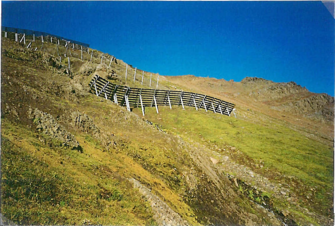
Photograph 3. Supporting structures from J. Martin, Geobrugg and EI in Hafnarfjall in Siglufjörður, northern Iceland.
