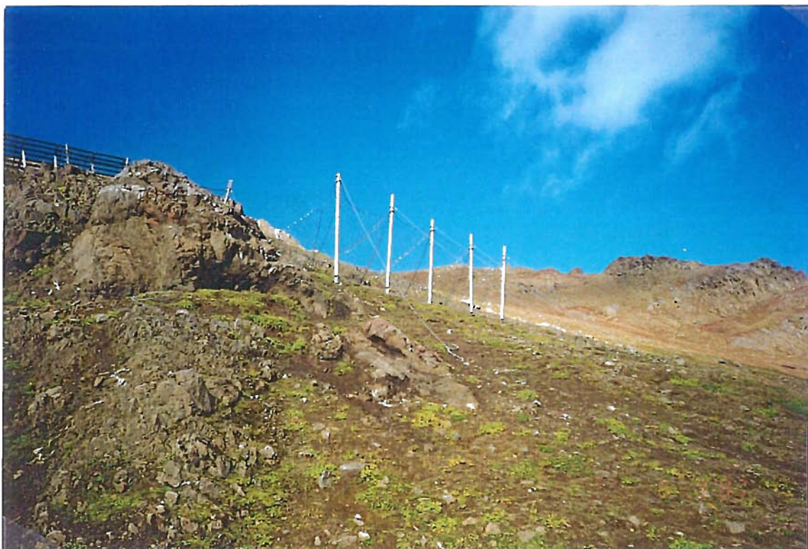
Photograph 8. A part of the EI nets in Siglufjörður showing a net which has been pulled down along the perimeter wire ropes.
