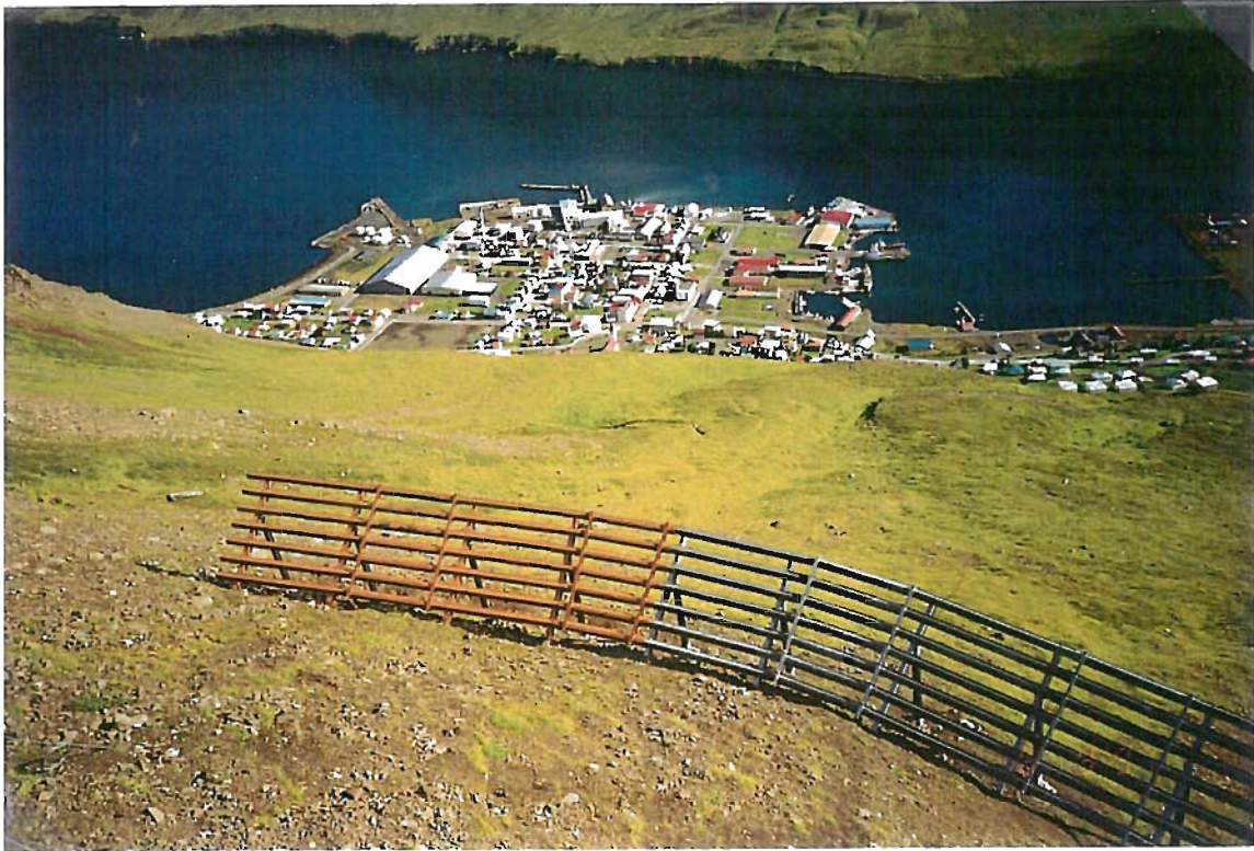
Photograph 5. A part of the stiff steel structures from J. Martin in Siglufjörður showing both black and galvanised bridges.
