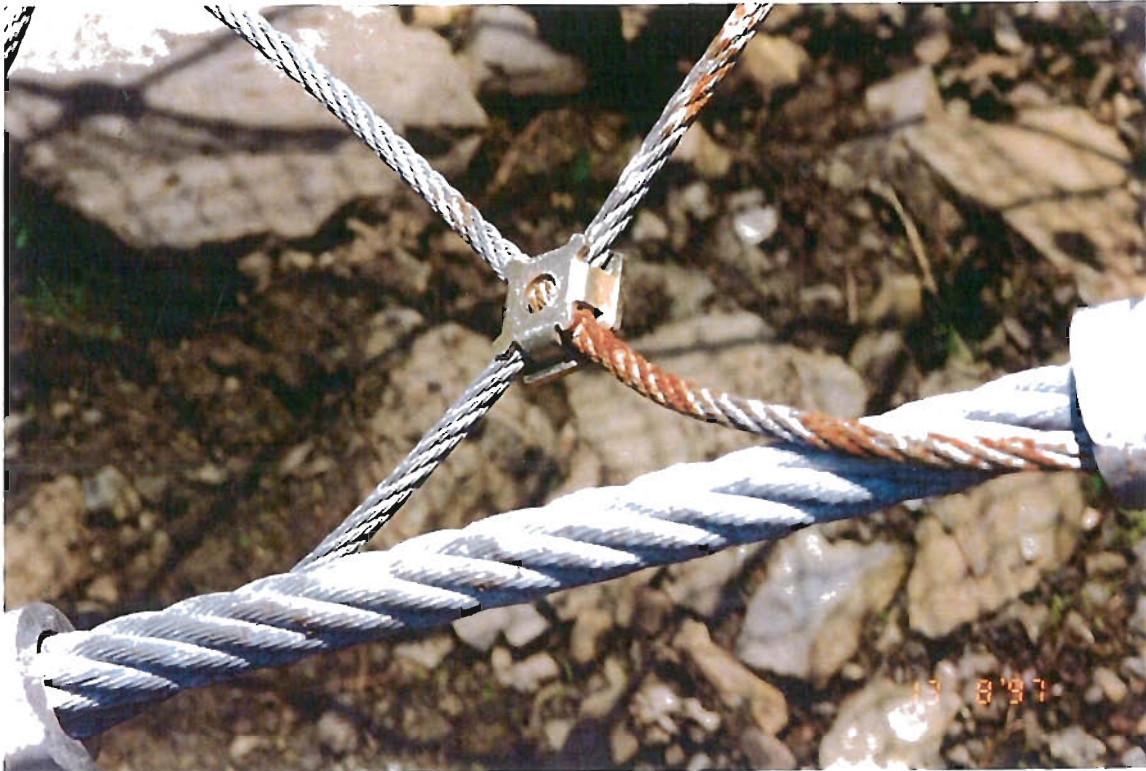
Photograph 7. Rusty clips and wires from the Geobrug nets in Siglufjörður.
