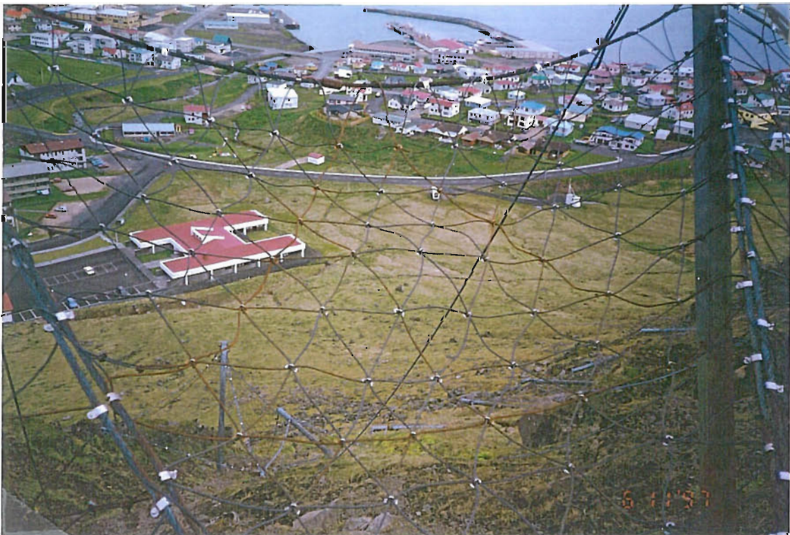
Photograph 4. A rusty part of the EI nets in Ólafsvík.
