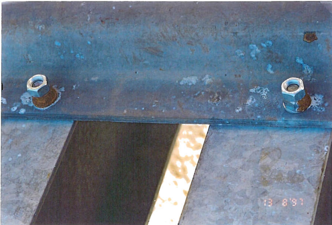
Photograph 6. Rusty nuts and bolts in the steel bridges from J. Martin in Siglufjörður.
