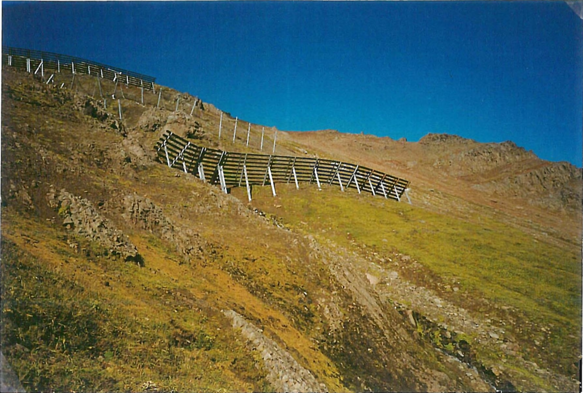
Photograph 1. The supporting structures in Hafnarfjall in Siglufjörður, northern Iceland.
