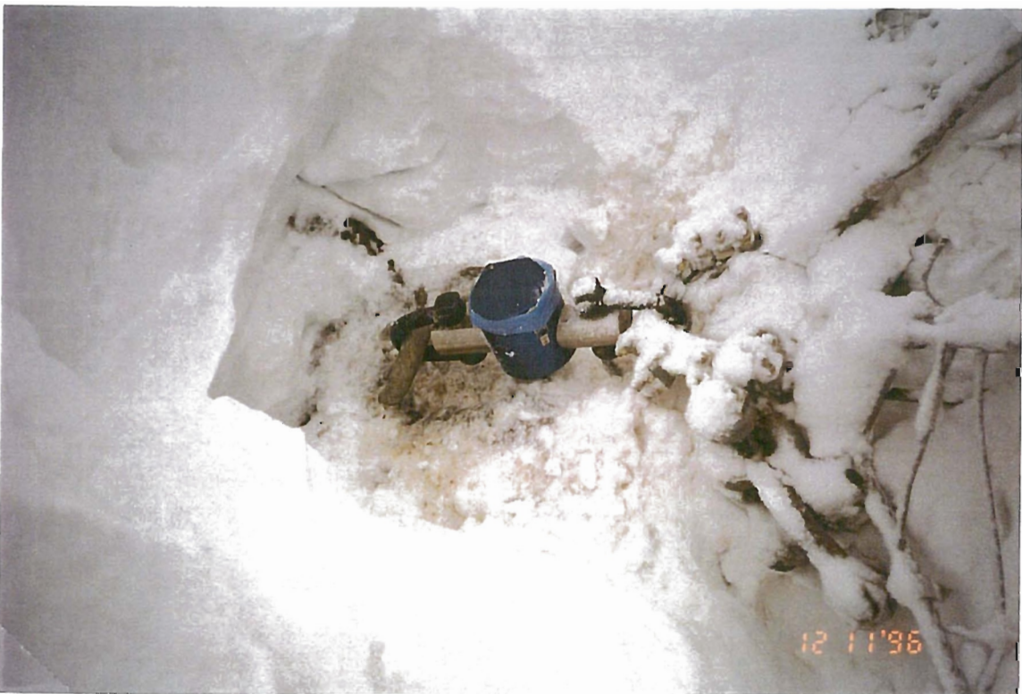
Photograph 2. The tension recording instrument in the Geobrug nets in row II.
