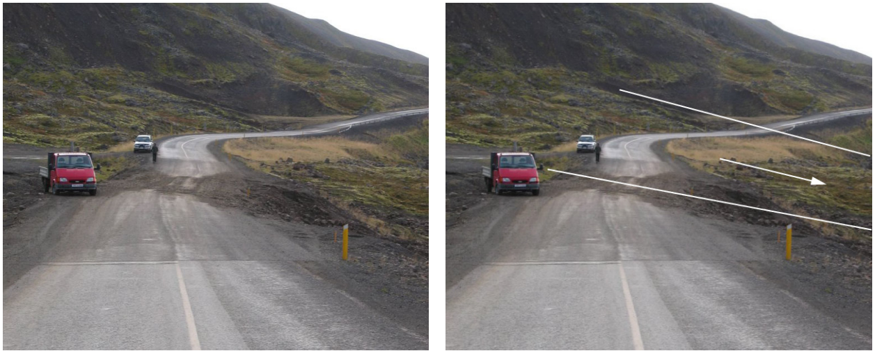
Figure 12. Looking south along the road from Siglufjörður town in Almanningur exhibiting meter-scale displacement of a portion of the road since its surface was paved.
