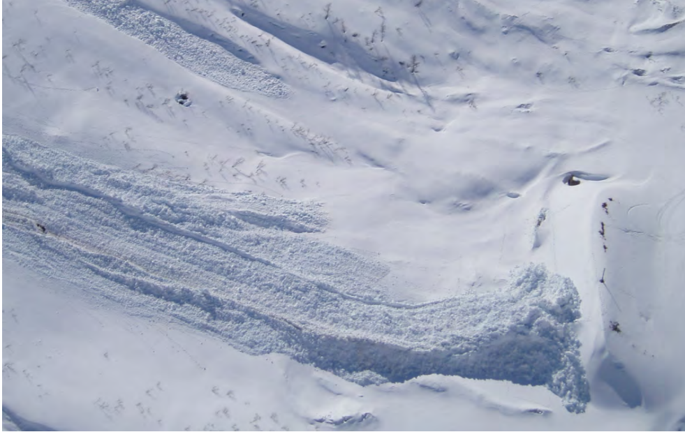
Figure 19: A wet-snow avalanche stopped by a catching dam in Ryggfonn, western Norway, on 16 April 2005, photograph: NGI.
