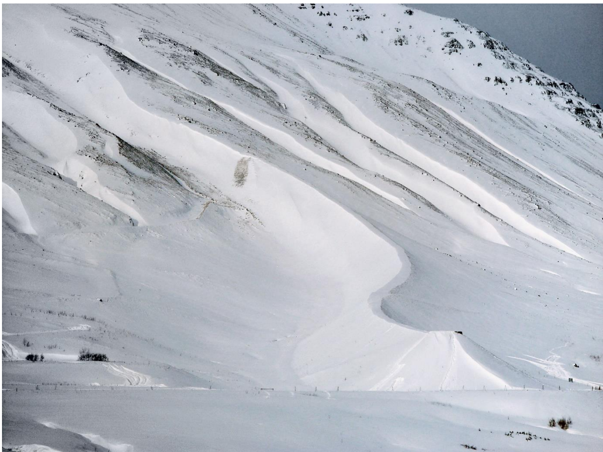
Figure 7 Stóri-Boli, deflecting dam in Siglufjörður, N-Iceland.
