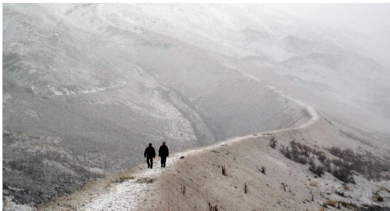
Figure 3 Stóri-Boli, deflecting dam, in Siglufjörður, N-Iceland. An informal path to the mountainside.
