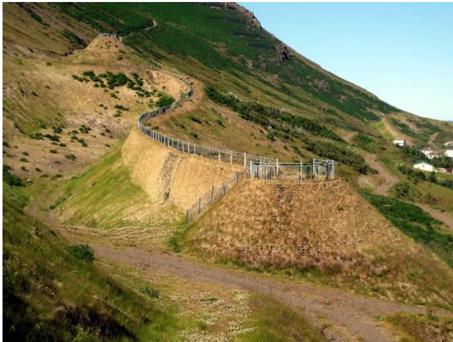
Figure 2 Catching dams above the town of Siglufjörður, N-Iceland. The ends of the dams are formed like sloping bastions with a public viewpoint.
