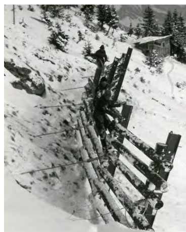
Figure 6: "Snow-hanging bridges", D_k = 3\text{m} , mounting after snowfall in the 60s of the last century in the avalanche starting zone of the Hüggen avalanche [Source: WLW Vorarlberg]
