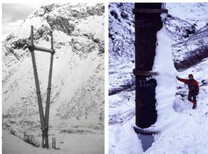
Figure 2 Avalanche impact on a circular cylinder tower. Photo by NGI
