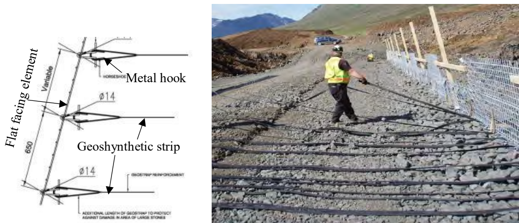
Figure 4 System no. 3: Flat facing panels. A schematic diagram, with units in mm, and a photograph during construction in Neskaupstaður.
