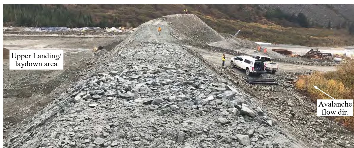
Figure 2 Construction of the deflection berm with temporary access ramp (October, 2018).
