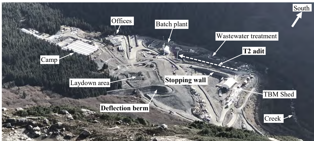
Figure 1 Horetzky Landing, viewed from the start zone of avalanche path 28.0N during late-stage construction of the deflection berm and stopping wall (Photo: October, 2018).
