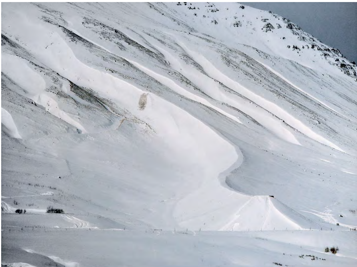
Figure 7 Stóri-Boli, deflecting dam in Siglufjörður, N-Iceland.
