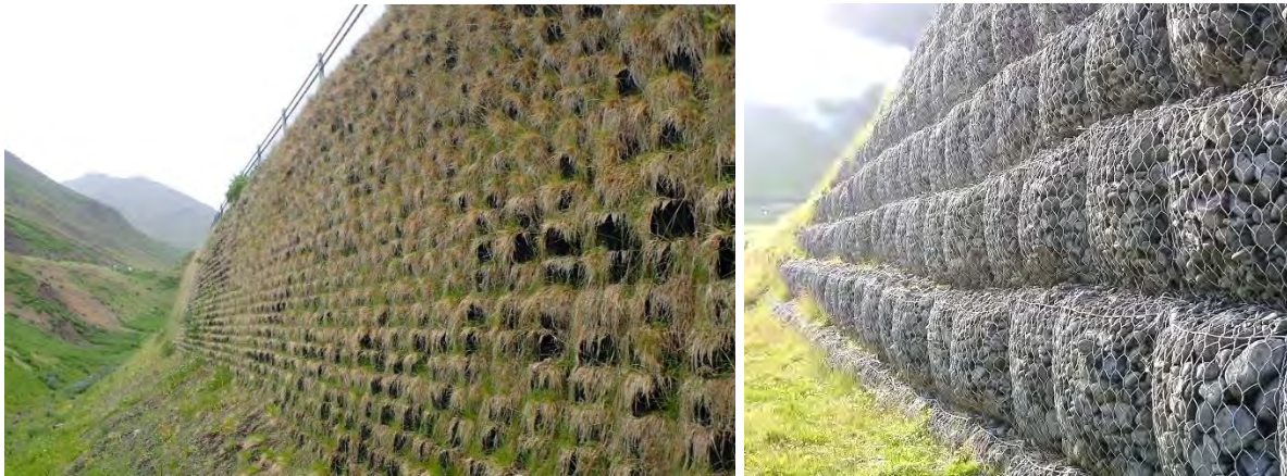
Figure 9 System no. 4, on the left, an example of final appearance in Siglufjörður. System no. 5 on the right, an example of final appearance in Ísafjörður. The fill material is rounded gravel.
