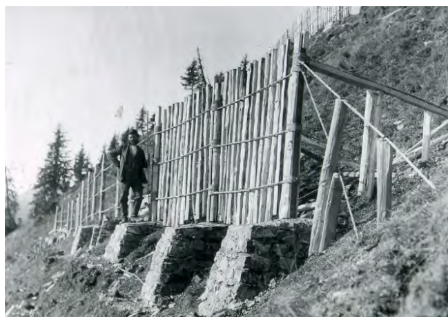
Figure 5: Arlberg Rake in the avalanche starting zone of the Hüggenlawine in the year 1906 [source: WLW Vorarlberg].
