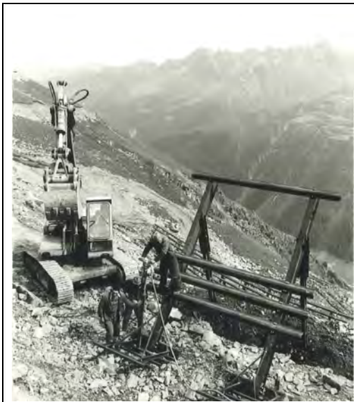
Figure 1: Installation of a supporting structure with a height of 3.5 meters, the foundation will be fixed with a concrete base and will be filled with soil material.
