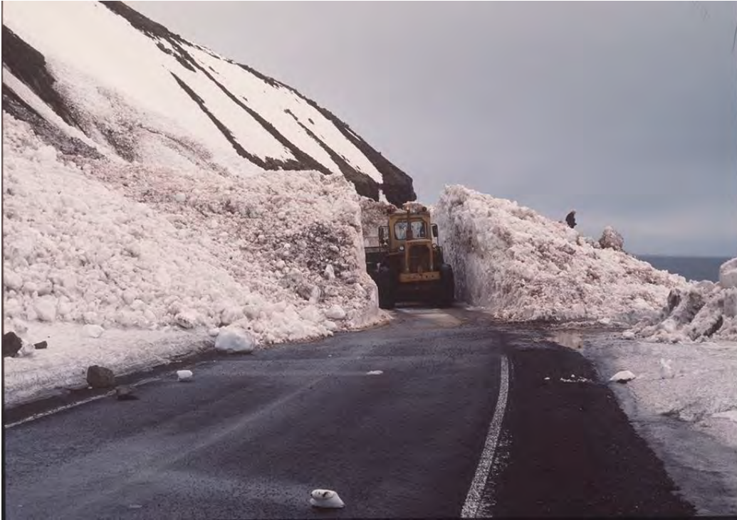
Figure 7. Clearing of an avalanche on road 61 at Óshlíð. The road was replaced by a tunnel in 2010.
