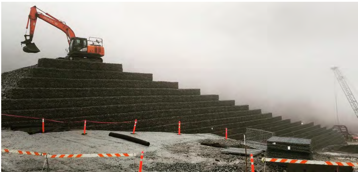
Figure 3 Final construction of the avalanche stopping wall (November, 2018).
