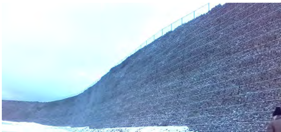
Figure 8 System no. 3 – an example of final appearance in Ísafjörður.
