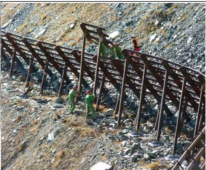
Figure 5: Construction Type flexible
