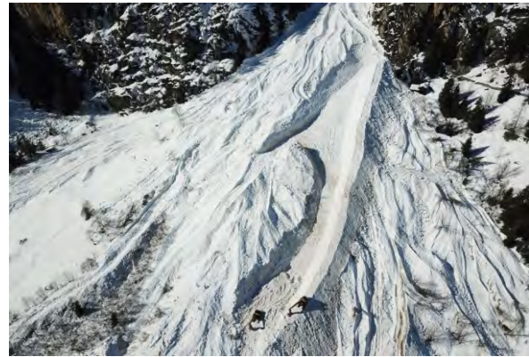
Figure 6 Deflecting dam made of snow, canton Valais (Photo W. Gitz, 2018)
