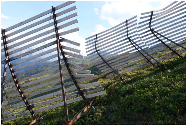
Figure 5 Snow drift fence damaged by lateral snow pressure acting in the line of slope, Valtschamela, canton Grisons (Photo S. Margreth, 2018).
