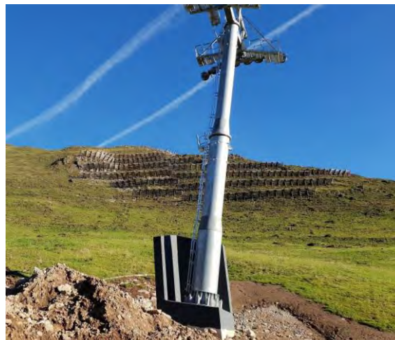
Figure 4: Elevated and wedge-shaped foundations to protect the pylons against flow avalanches (KitzSki, 2019)
