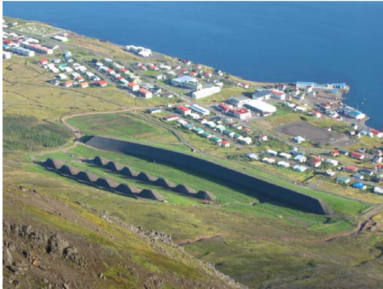
Figure 2: A photograph of the braking mounds in Neskaupstaður and the catching dam behind them. Each mound is 10 m high and the catching dam is 17 m high.
